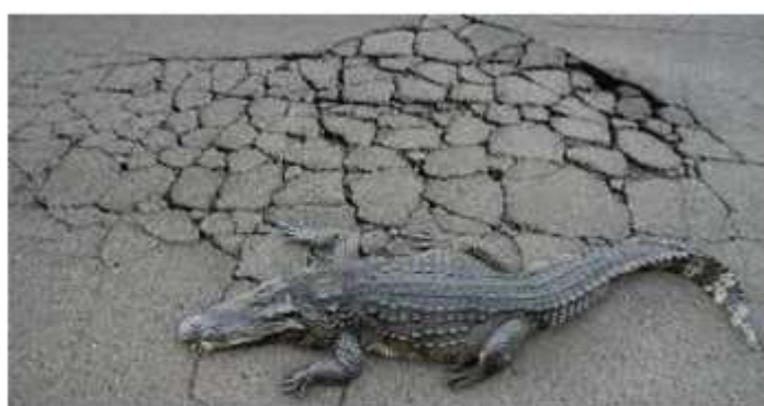
CROCODILE CRACKING OF ROAD SURFACE
